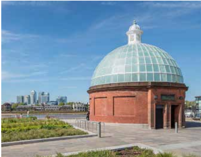
The refurbished south rotunda close to the Cutty Sark at Greenwich. A separate entrance was provided for people using the lift and the stairs. The plaque illustrated above is seen above the entrance doorways. Photo by Diliff
